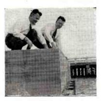
M. C. SCOTT (1), chief engineer, WIOD Miami, Fla., explains to J. Leonard Reinsch, managing director, Cox stations, details of the construction of a concrete anchor for one of the new hurricane-proof towers being built at WIOD's transmitter site in Biscayne Bay. Total weight of the concrete and steel in the three anchor foundations and the tower base foundation is 3,527,000 lbs.
